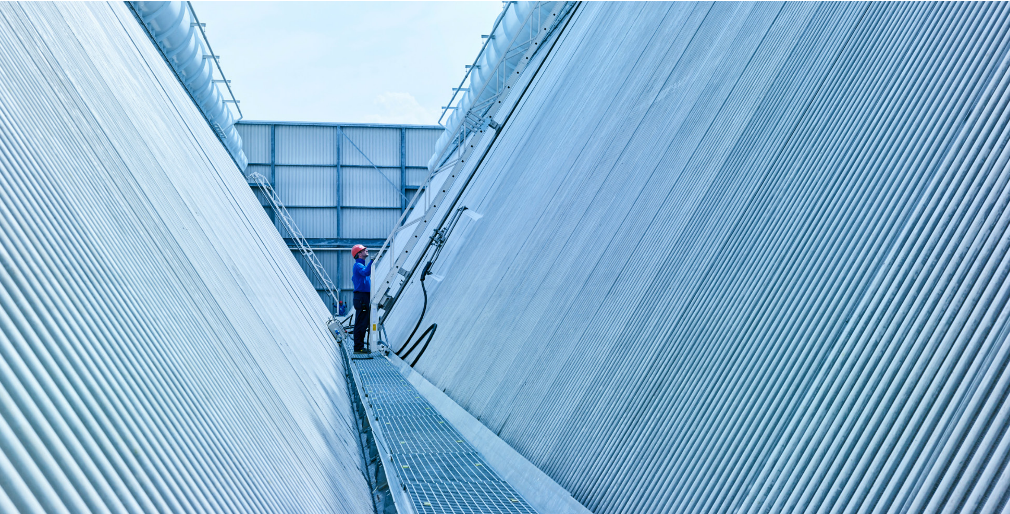
Cooling system in the Livorno Ferraris power plant
