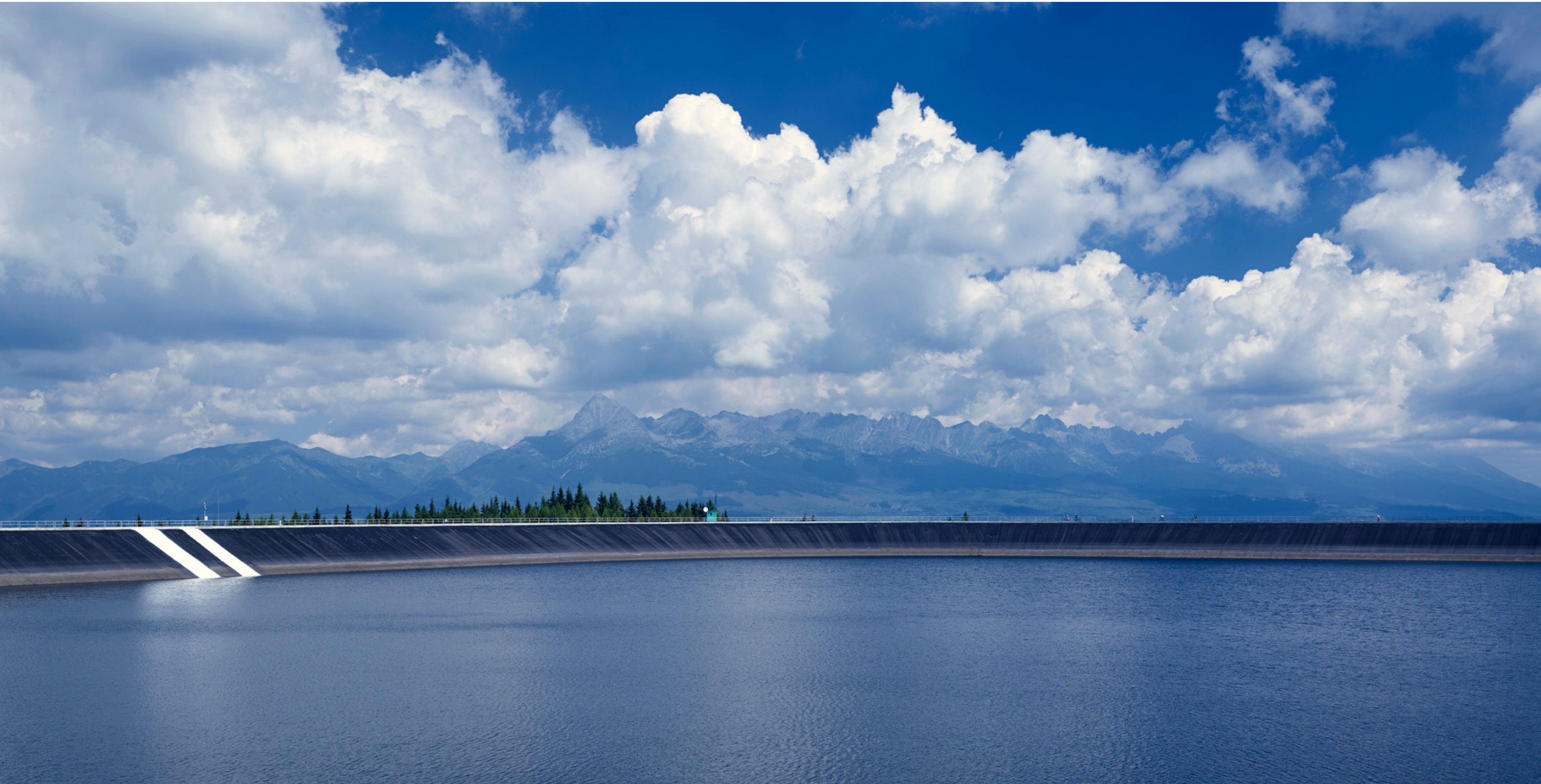
The upper reservoir of the Čierny Váh pumped-storage hydroelectric power plant
