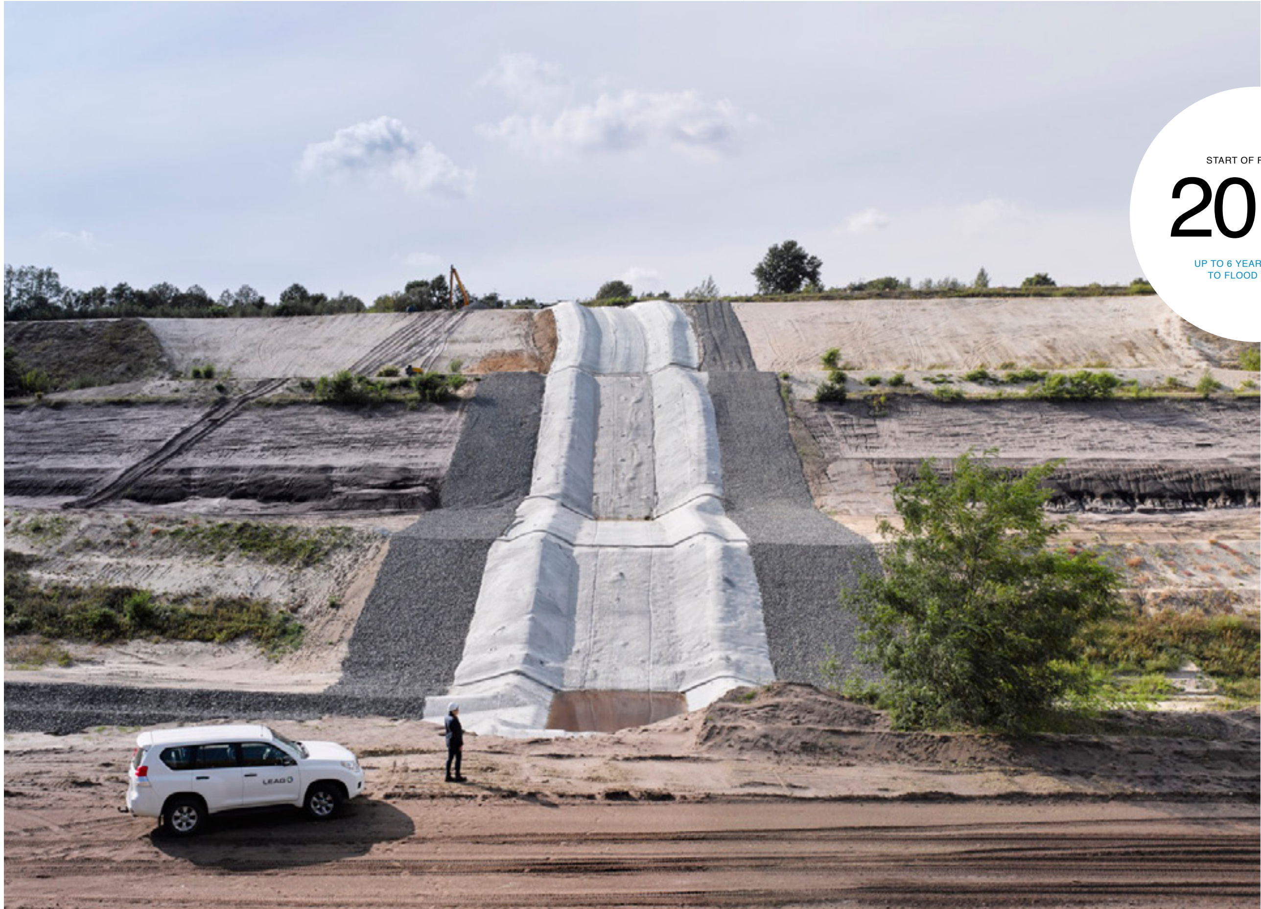
Fig. 72 LEAG is preparing lake bed and slopes for Cottbuser Ostsee, so that gradual flooding from the Spree River can start by end of 2018.
