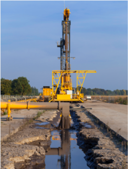
Picture 16: To construct an underground sealing wall, the digging tool cuts through the soil layers. It creates a one-meter wide slot. This slot is filled with a clay-water mixture. Due to the hydraulic overpressure in the slot the water molecules to pass outward leave a clay filter crust over at the side walls of the slot, ensuring a water-impenetrable barrier. Finally, the slot is backfilled with soil and the surface is greened.
