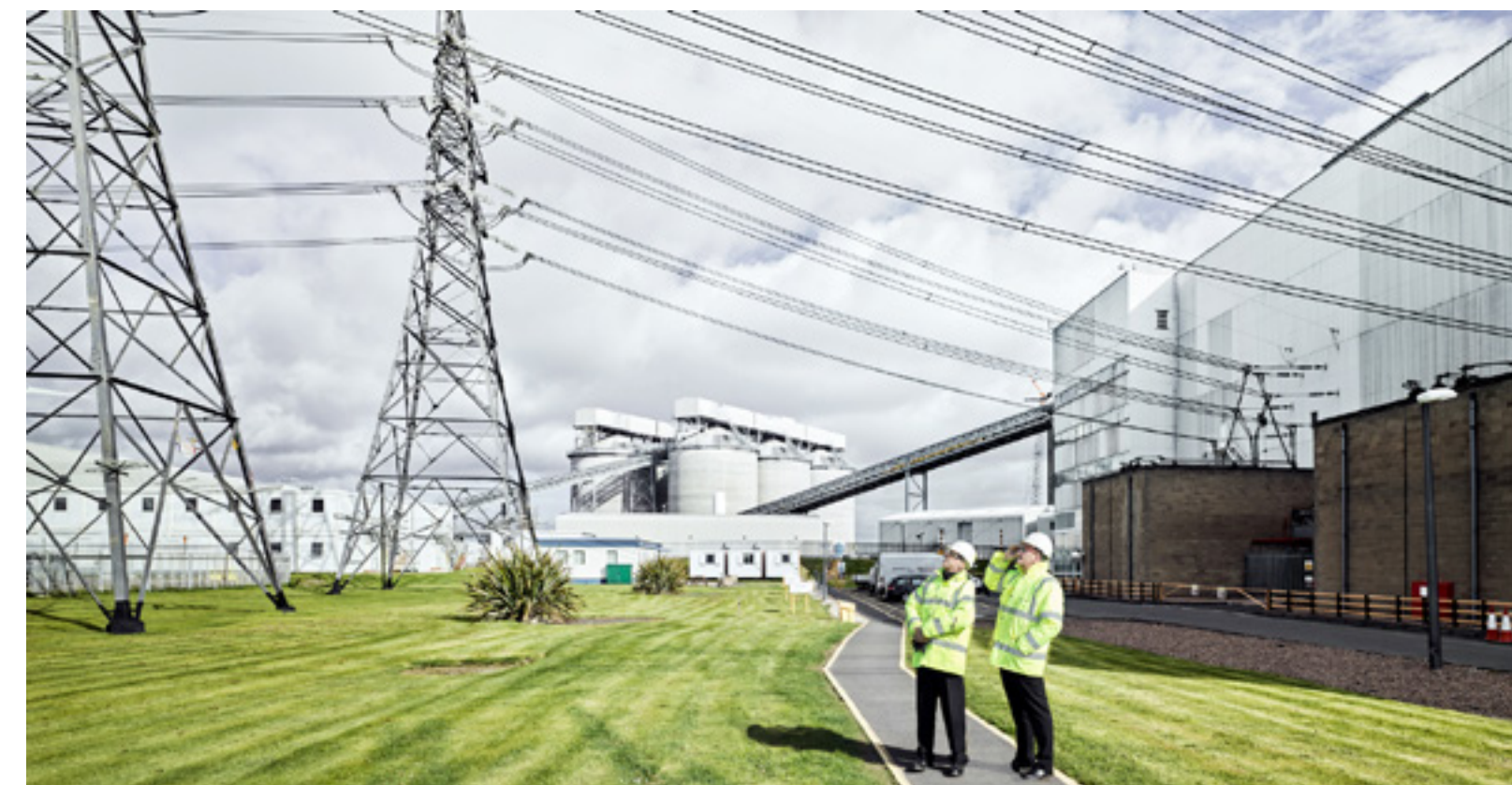
61 Lynemouth biomass power station.
