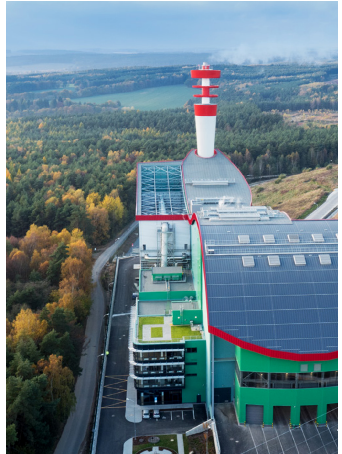
59 Waste combustion plant in the Pilsen region which is a part of Plzeňská teplárenská a.s.
